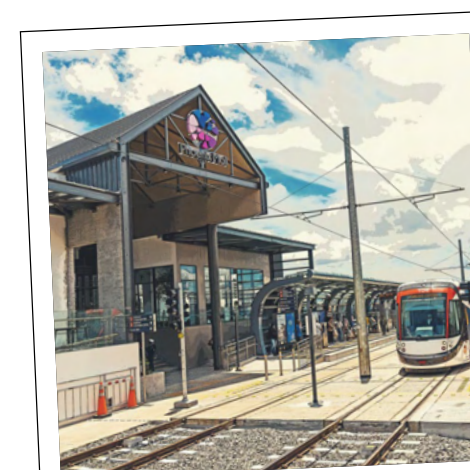
Completion of Phoenix Mall Station
