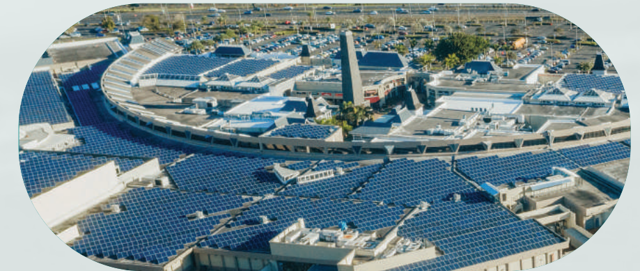
PV Farm at Bagatelle Mall
